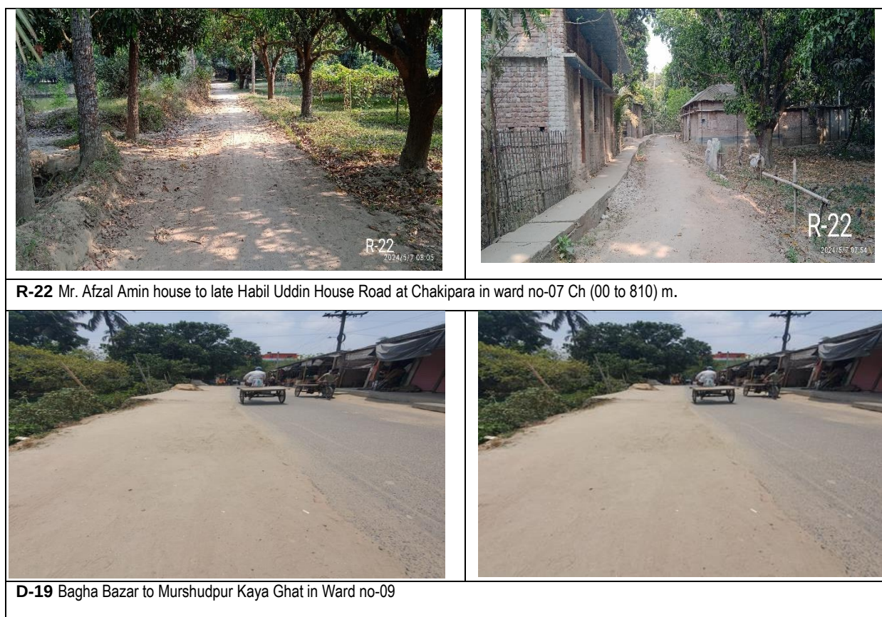
Figure 4:Existing Roads and Drains Picture
